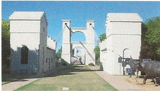
Historic Suspension Bridge on Brazos River
